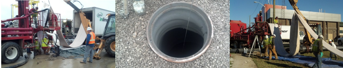
ALL: Construction Photos of Lining Operation and Manhole Restoration
