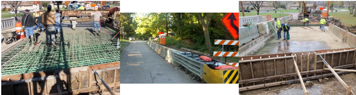
Construction Photos Bridge Work
