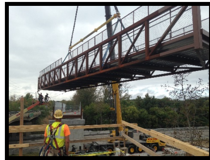
Setting Pedestrian Bridge Span Over I-74
