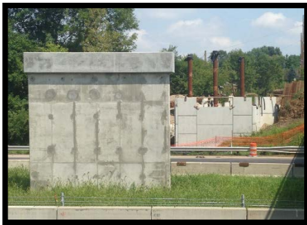
Construction of Pedestrian Bridge Piers
