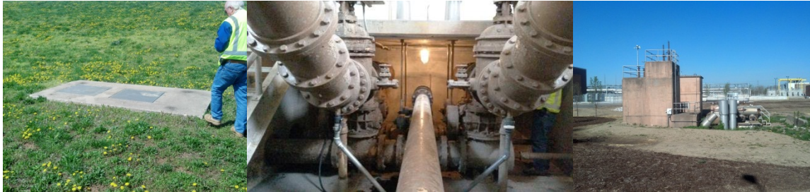
Drainage or Air Release Valve Structure on Concord Street
